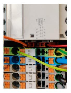
b. Mount the cable tie for strain relief on the charging cable after it enters the M32 cable gland.
